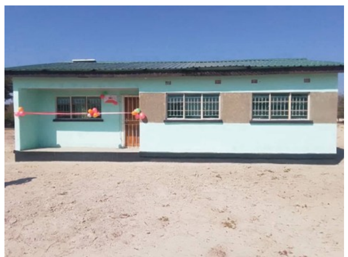
Constructed teachers accommodation
