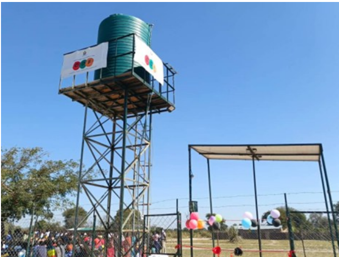
Commissioned water tank project with solar panels
