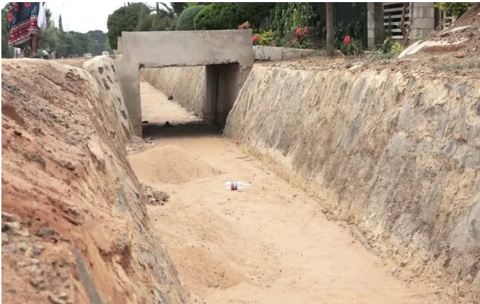
Newly built drainage channels
