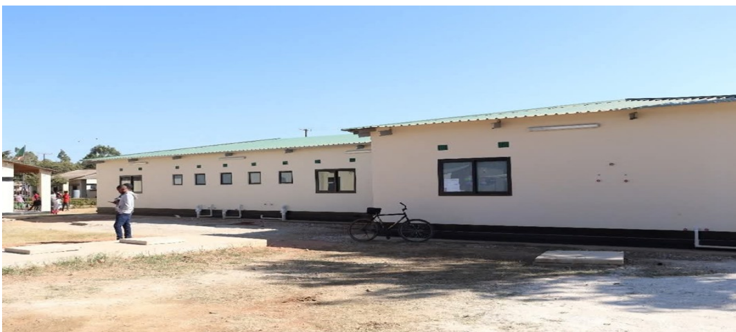
On the left—Newly constructed maternity ward.
