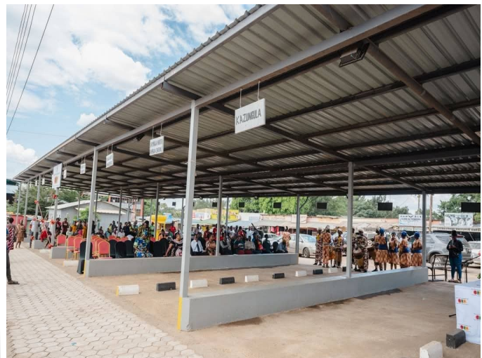
Newly constructed taxi rank shelter
