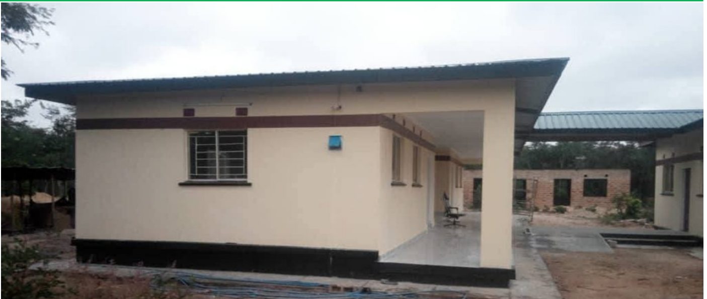
The newly commissioned Kanchibiya mothers shelter.
