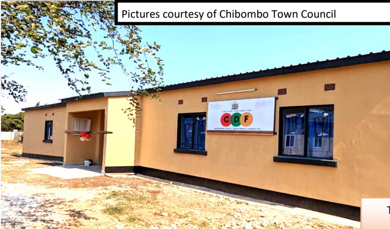
The newly constructed Mwanjuni Maternity Wing in Katuba Ward.
