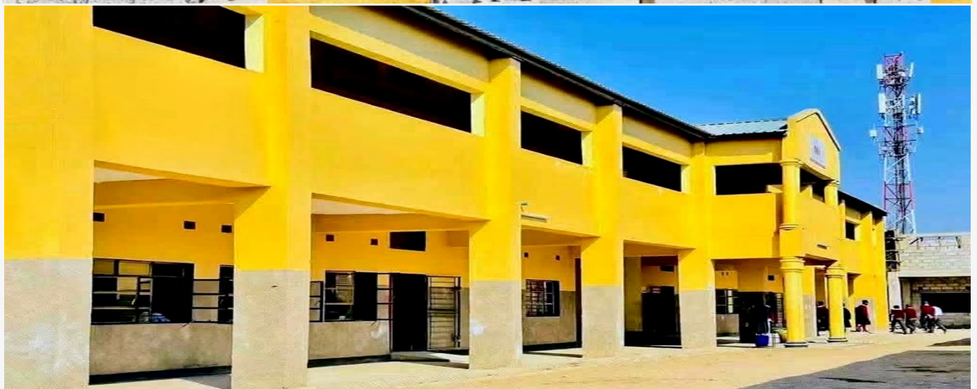
The newly constructed double-storey 1x6 classroom blocks in Chawama, Kanyama and Bauleni constituencies in Lusaka.
