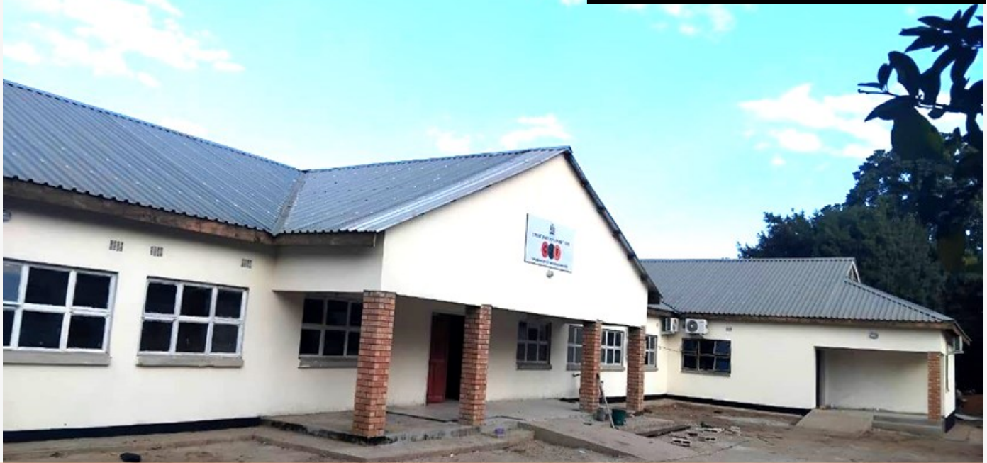
Linda Mini Hospital in Nansanzu Ward nears completion under the 2025 CDF.
