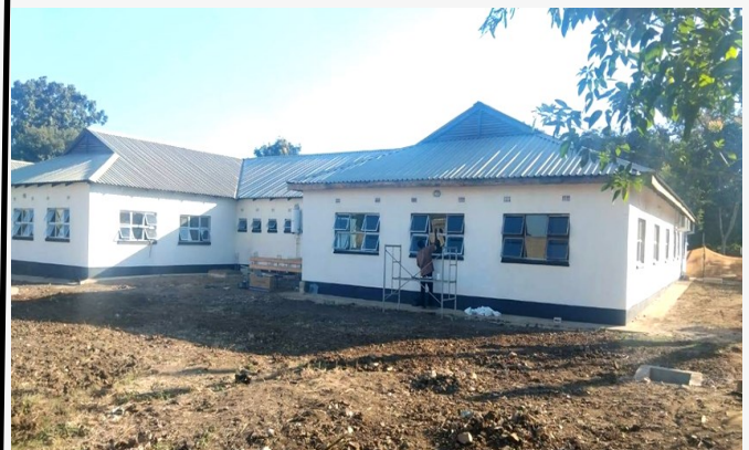
Final finishing works underway at Linda Mini Hospital
