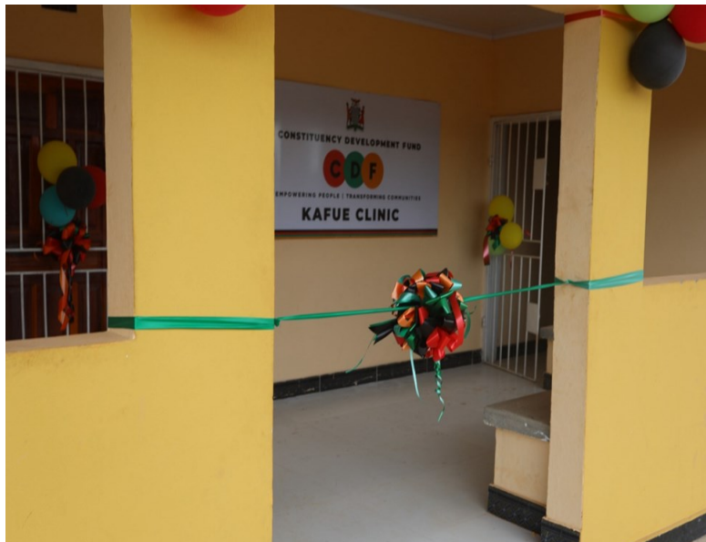
A newly constructed Standard Health Post at Kafue Park Clinic in Kitwe
