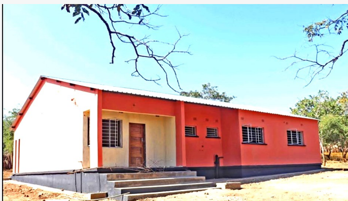
Newly constructed staff House at Mkale Health Post in Mkaika Constituency.
