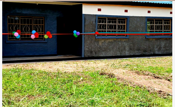
The solar-powered police staff house at Kankolonkolo, funded through CDF
