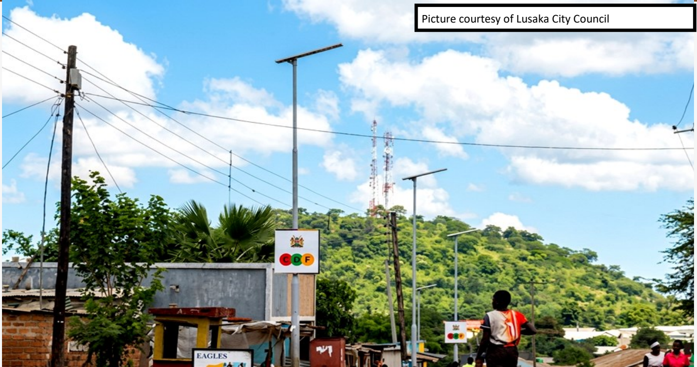
The newly installed street lights in Kanyama Constituency.
