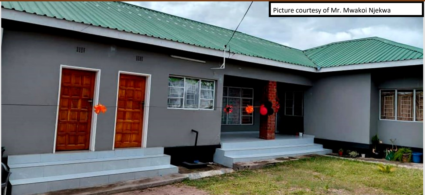
The newly constructed palace for Senior Chief Kandala of Limulunga District in Western Province.
