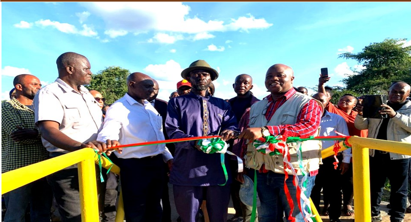
Central Province Minister and Katuba MP, Hon. Mwabashike Nkulukusa cuts the ribbon to officially handover the new footbridge in Chilochabalenje Ward.
