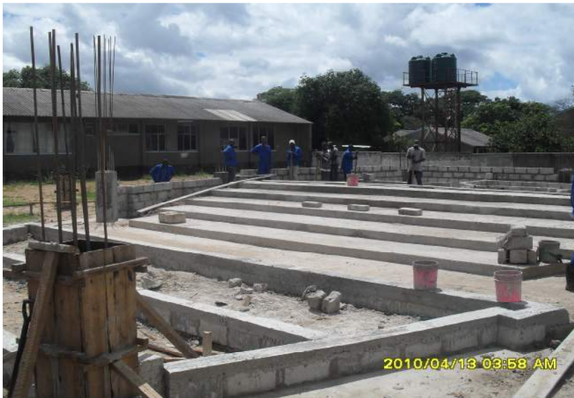
Construction of a Lecture Theatre at Kasama School of Nursing
