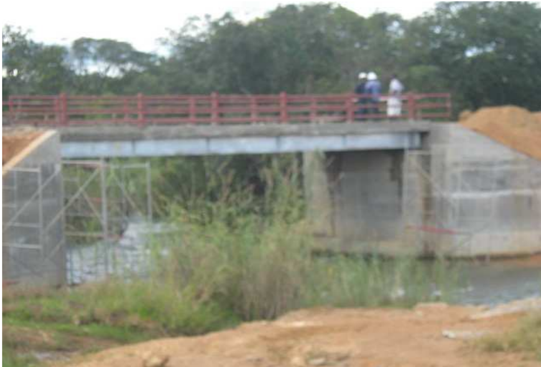
Part of the Luwombwa bridge being constructed in Nansanga Farming Block
