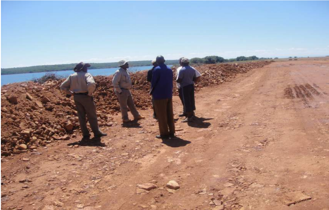
Part of the runway being constructed at Kasaba Bay
