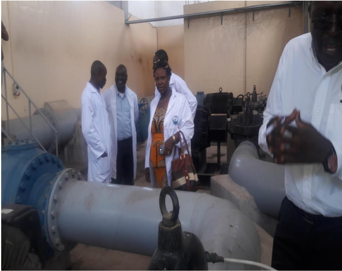
Mukobeko Water Treatment Plant – Lukanga Water and Sewerage Company
