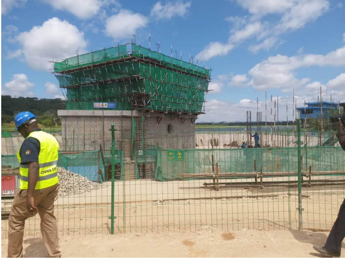
Kafue New Intake Treatment Facility – Lusaka Water and Sewerage Company
