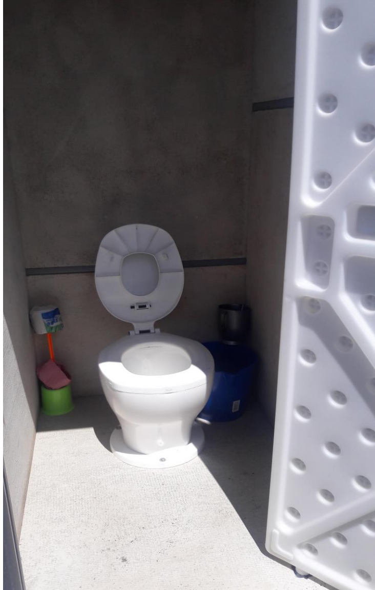
Eazi Flush Toilet Pilot Project - Lukanga Water and Sewerage Company
