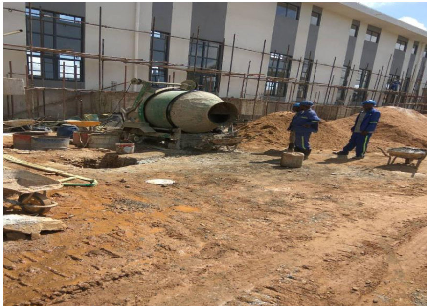
The Chilanga Booster Pump Station under construction
