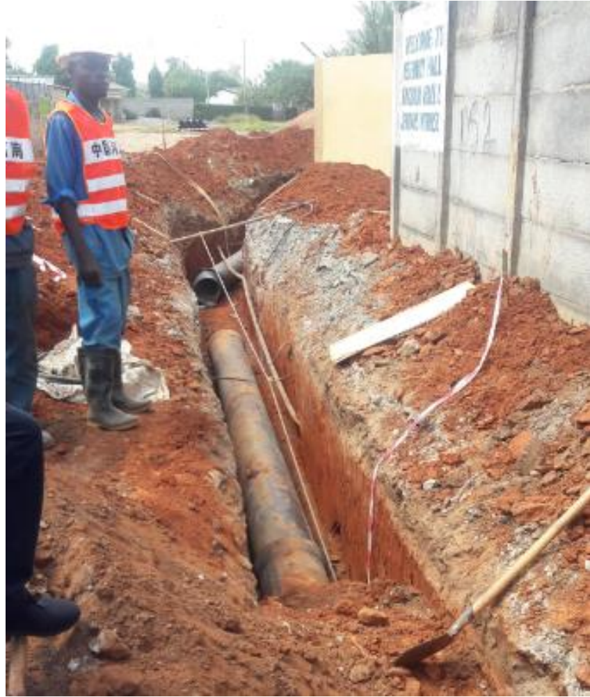
Installation of Ductile Pipes – Nkana Water and Sewerage Company
