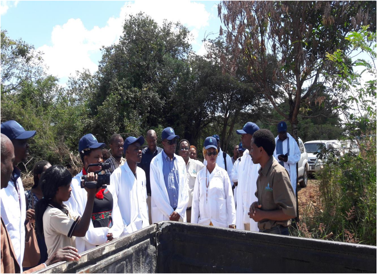
Members of your Committee at the construction site of the Kafulafuta Dam
