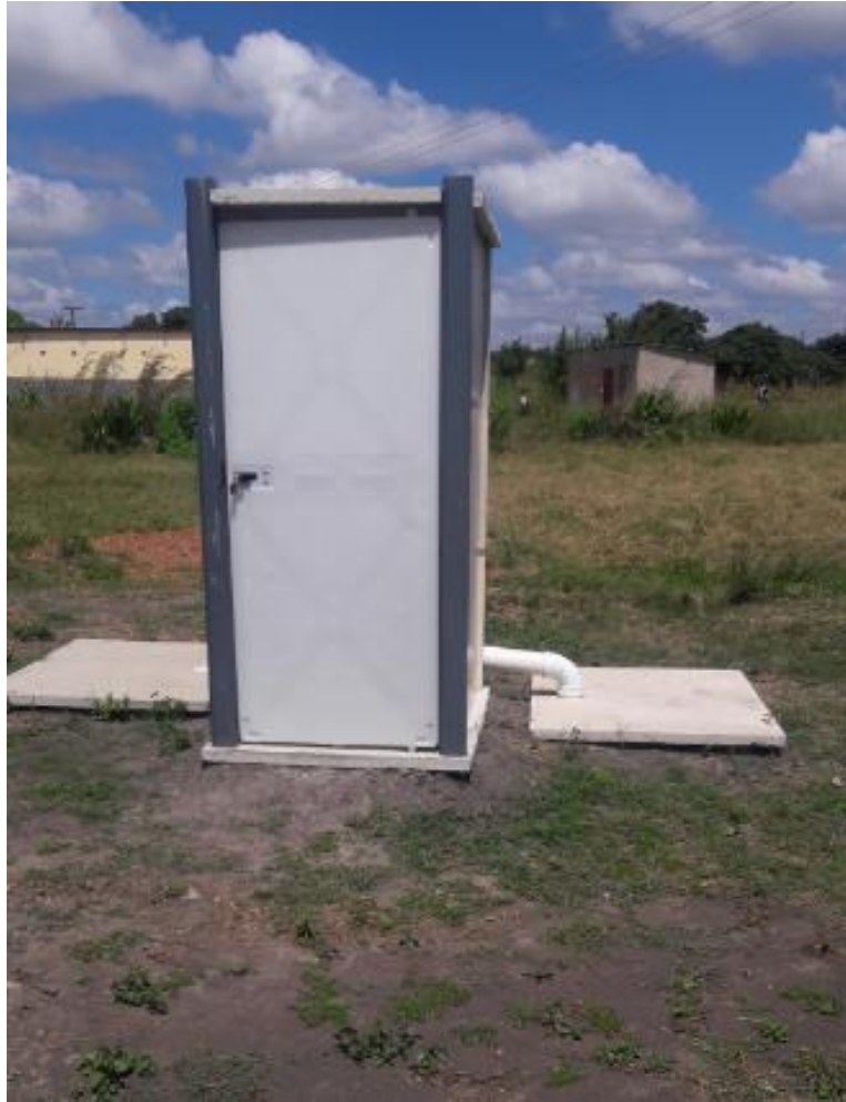
Eazi Flush Toilet Pilot Project - Lukanga Water and Sewerage Company
