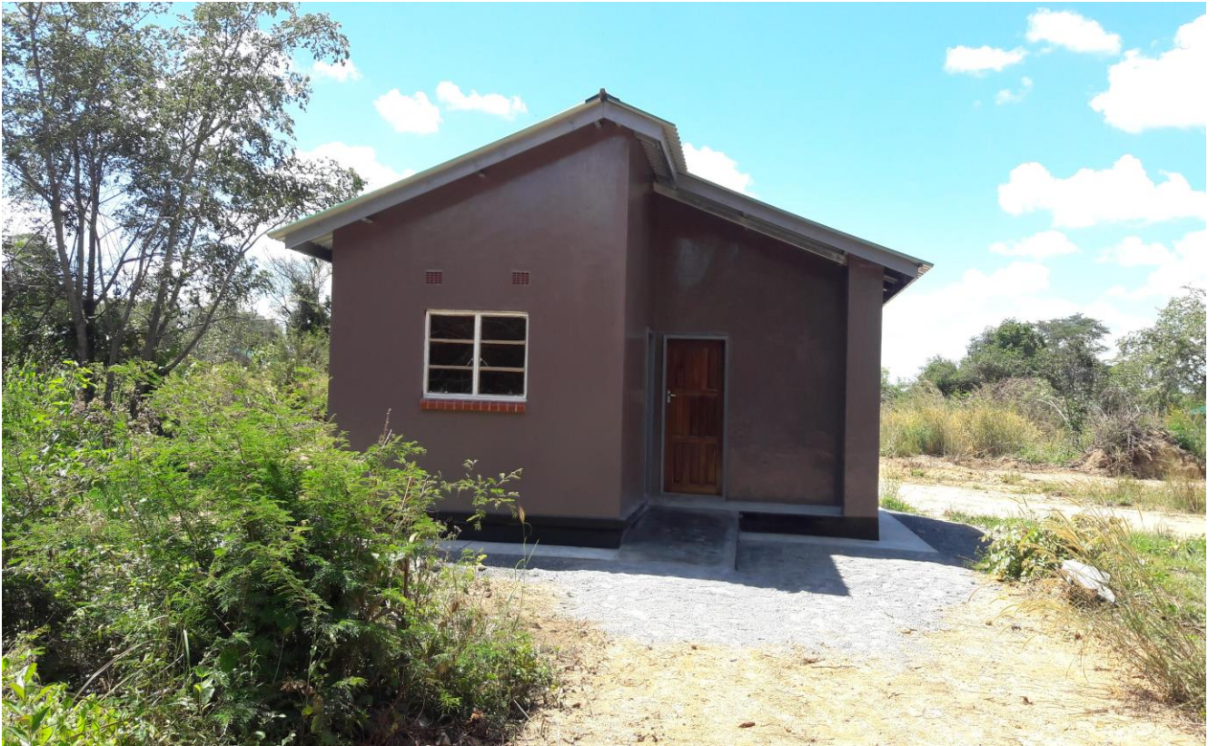
Kafulafuta Water Supply Scheme Project, Resettlement House
