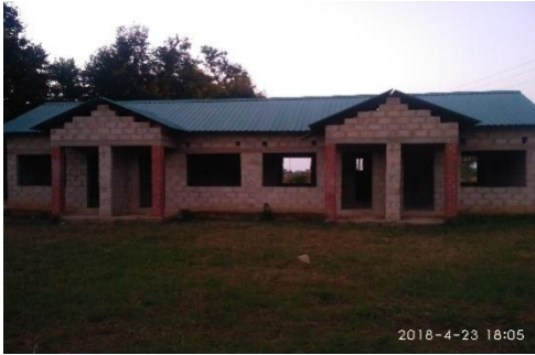
Uncompleted guest rooms at FTC – Monze
