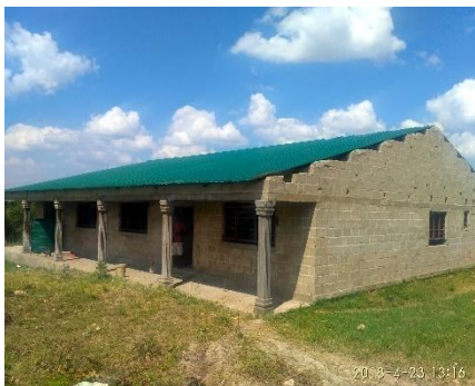
Uncompleted office block at Zimba
