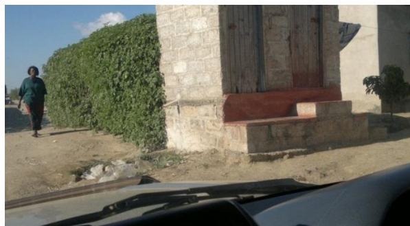
A toilet with waste water draining into a road
