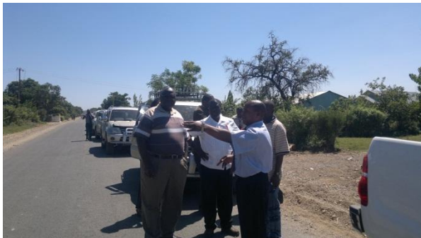
One of the township roads being worked on in Livingstone
