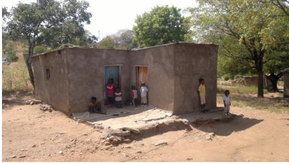
House under order of demolition in Mitcho
