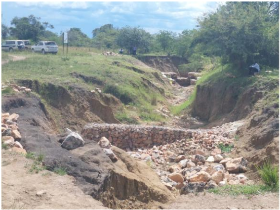
Mutama-Bweengwa River Headwater Gully treatment
