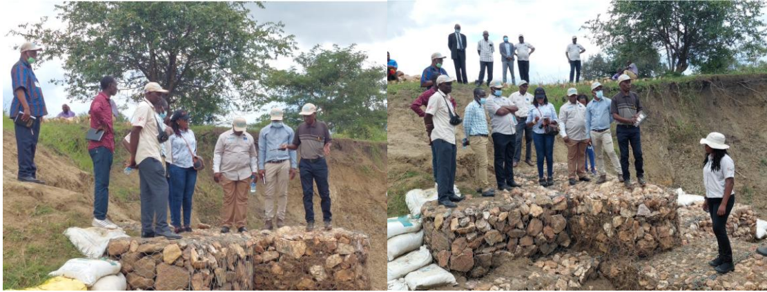
Water User Association Executive Member Mr. Likolo explains about the Check Dams
