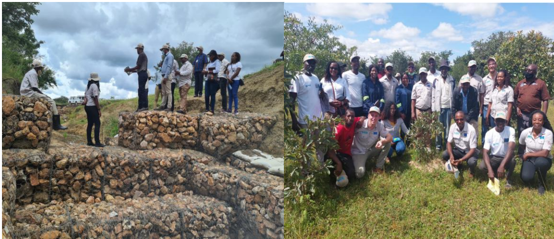
Gully erosion at Mweemba Musende site
