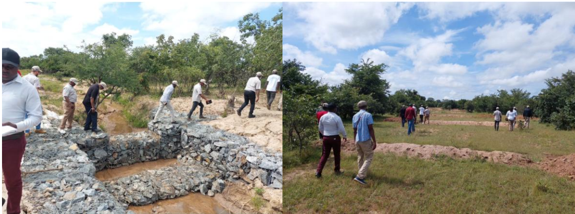
Check Dam at Mweemba Musende Catchment Protection Measure Site
