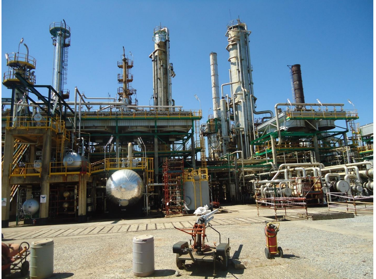
Part of the refurbished INDENI PLANT
