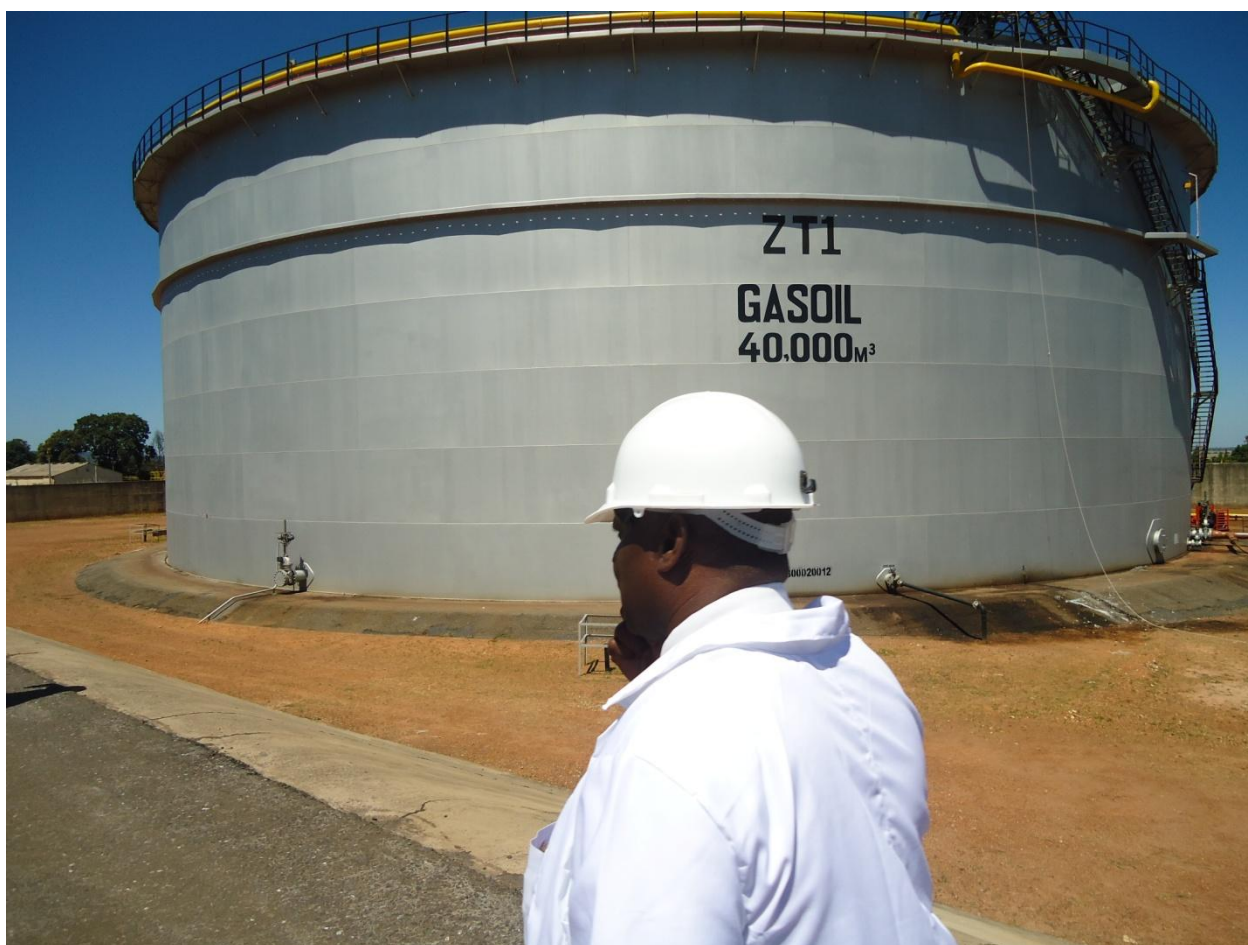
The recently rehabilitated ZT1 40, 000 m 3 tank at TAZAMA
