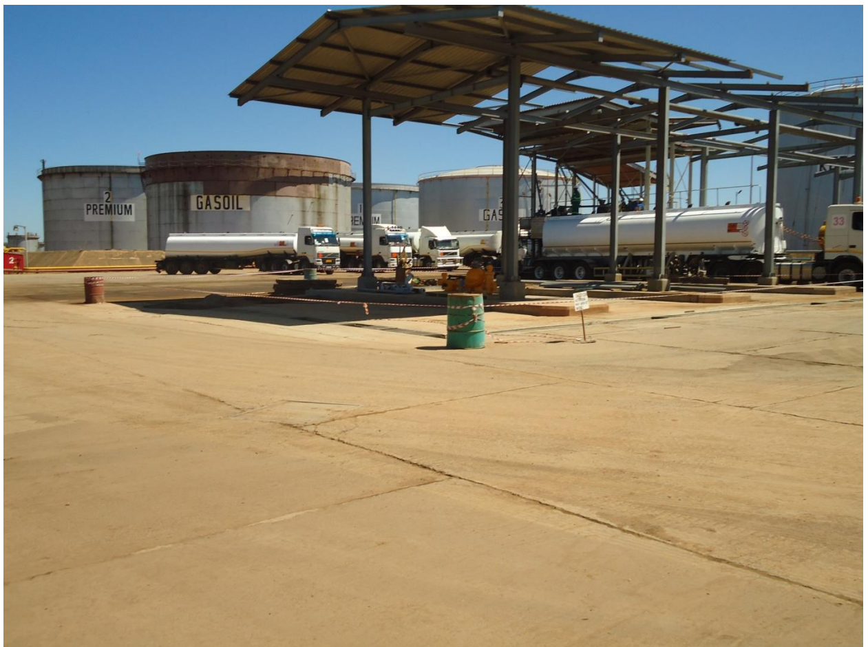
The Loading Bay and storage tanks at TAZAMA, which are under rehabilitation
