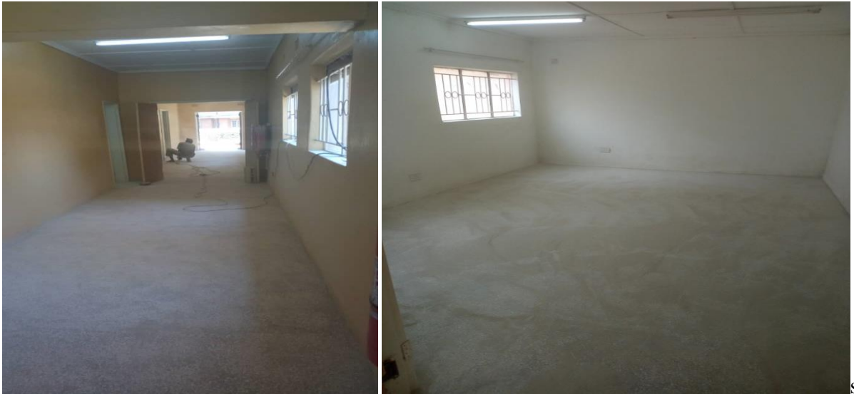
Fig: Contractor Levelling and Polishing the Terrazzo Floor.
