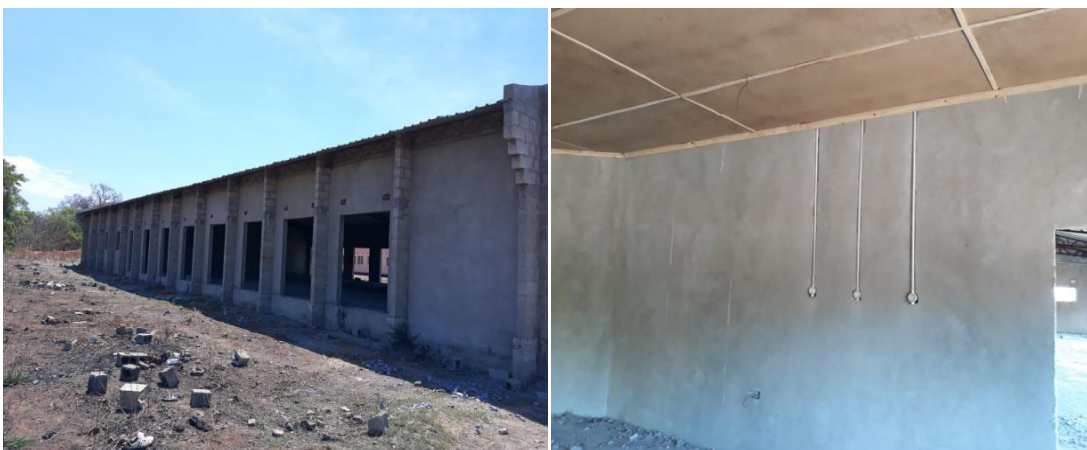
Fig: Showing External Plaster Works
