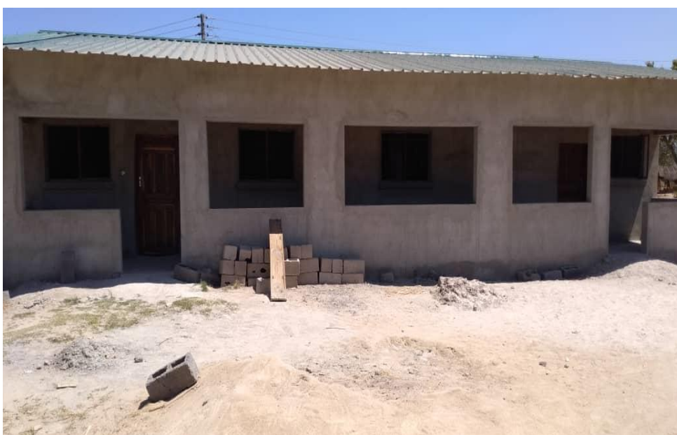
Fig: Showing Plastered Works to the Maternity Annex
