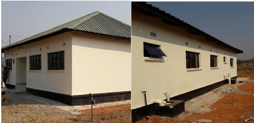
Current Status of Office Block as at 24/09/2019
