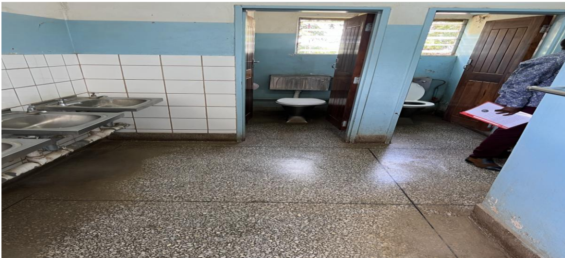
Toilets in the female ablution block
