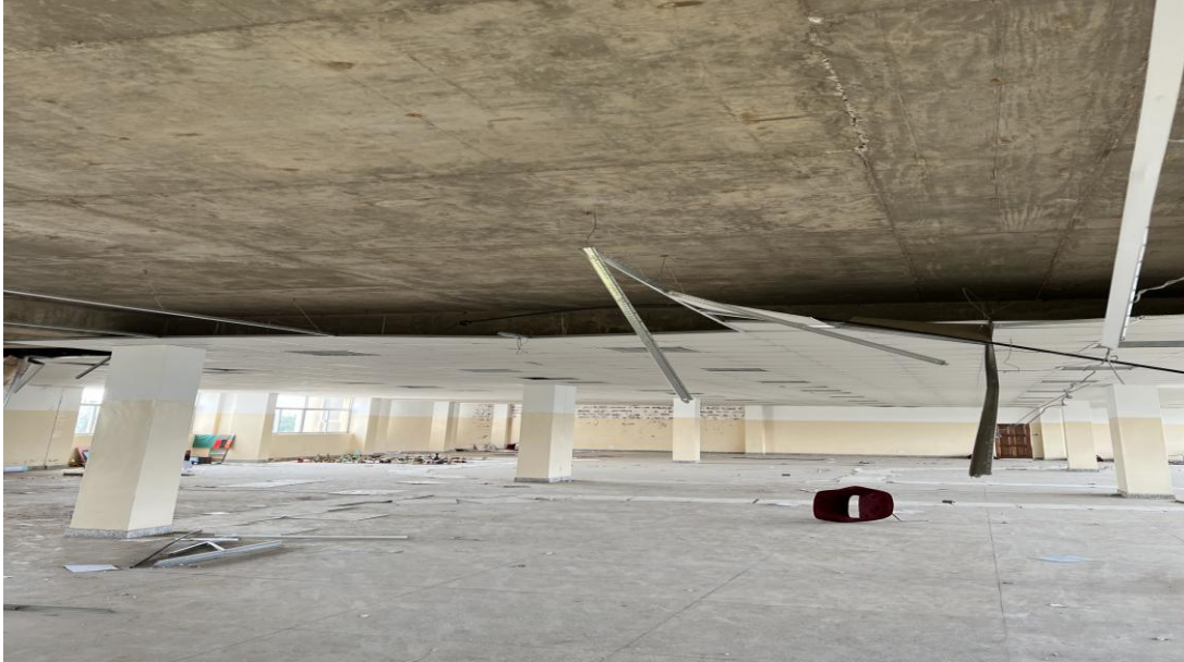
Part of the Ceiling inside the new structure
