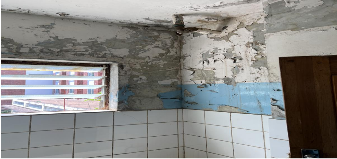
The walls in the female ablution block
