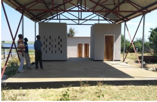
a) Fish freezing facility in Senanga – in progress
