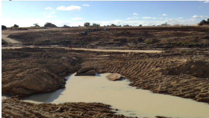
Fig. 25: Works at Mwomboshi Dam Site
