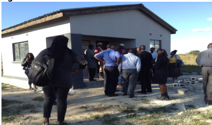
Fig. 26: Houses for resettlement at Mwomboshi dam
