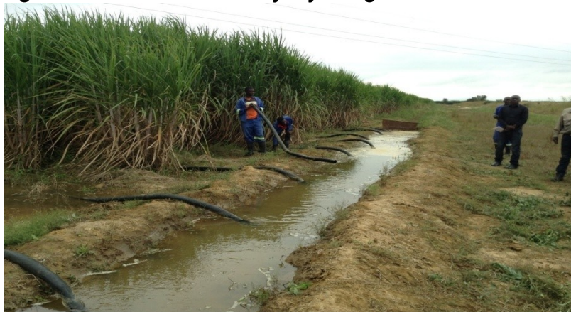
Fig. 1: Unlined canal at Manyonyo Irrigation Scheme
