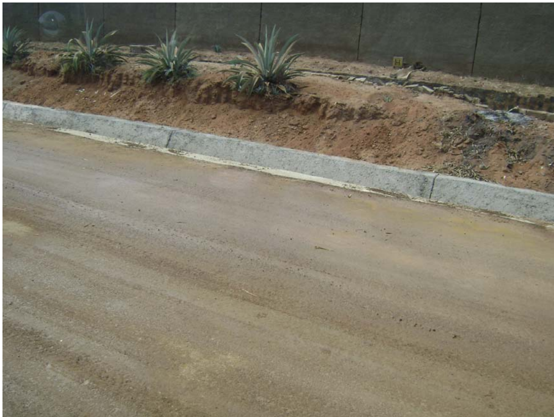
Rehabilitated Concrete Drainage - Livingstone
