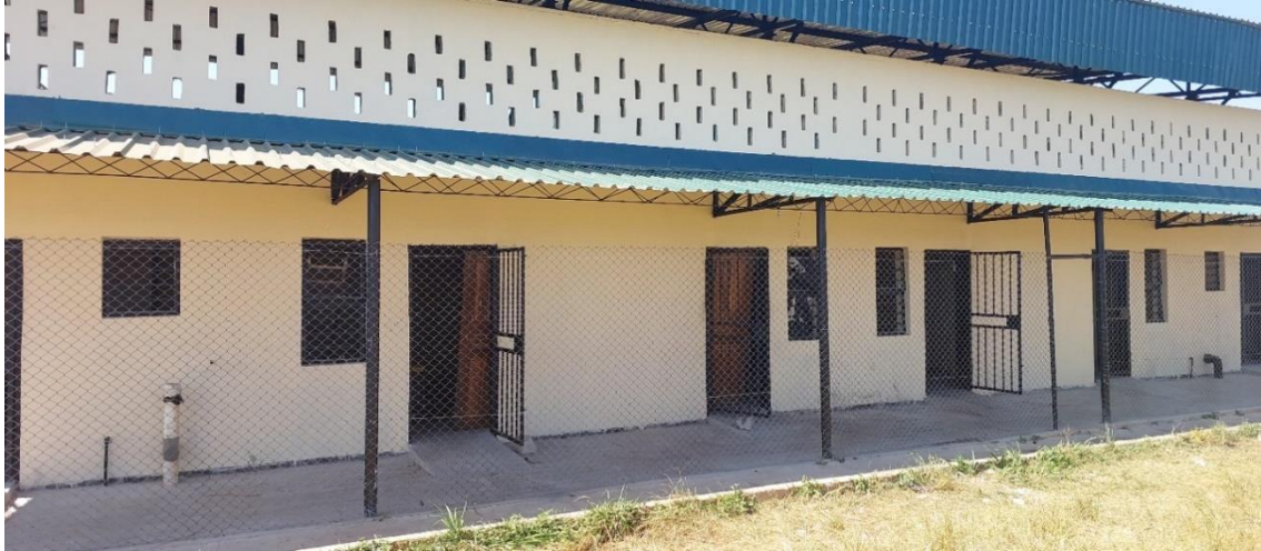
(i) Old dressing rooms under the grandstand being rehabilitated.
