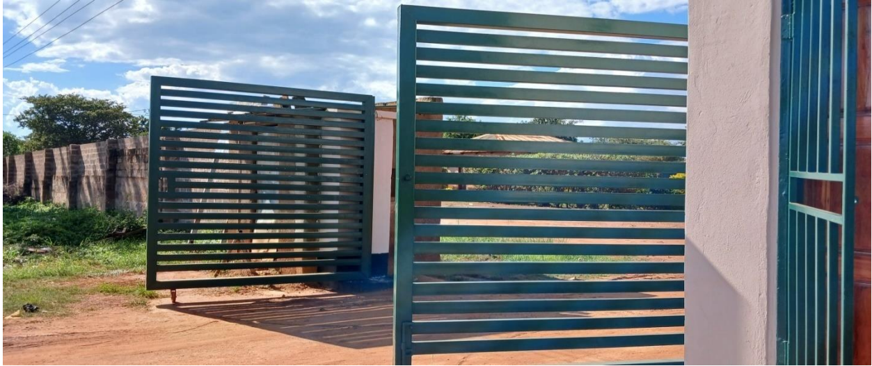
Figure (b) One of the newly installed steel gates
