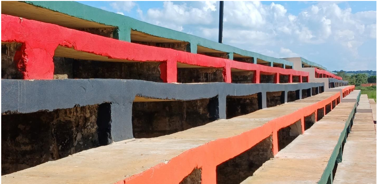
Figure (c) Terraces that are not well leveled
