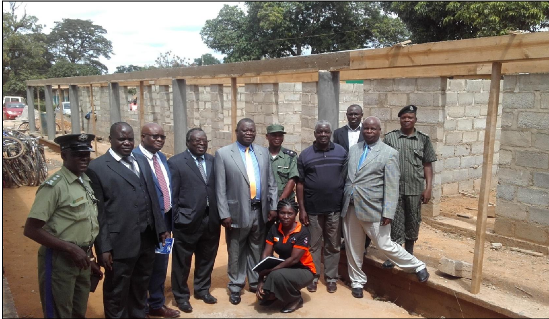
District Police Headquarters under construction on PPP in Mumbwa
