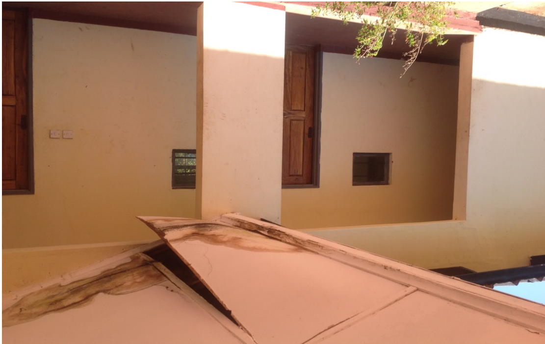
Picture 10: Rehabilitated Kabompo Guest House – Kabompo
