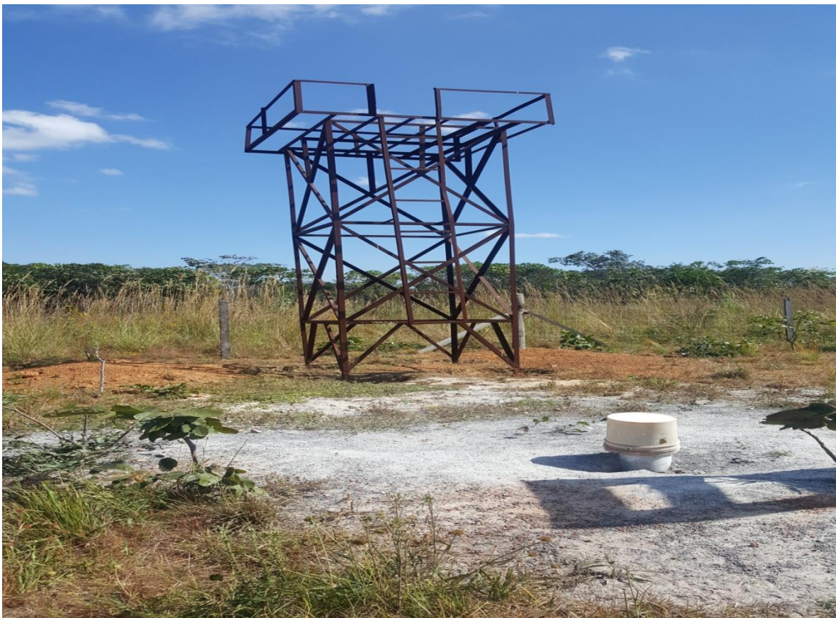
Fig.4: Incomplete Borehole Infrastructure at Luchembe Goat Breeding Centre
