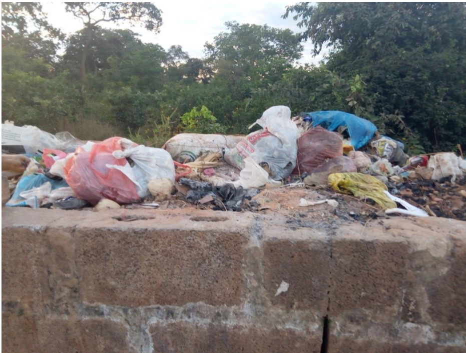
Fig.10: Perimeter wall of NRDC turned into dumping site by neighbouring compound
