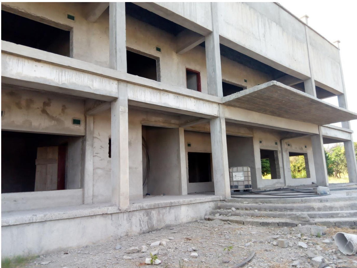
Fig. 13: Construction site for Ndola Regional Laboratory
