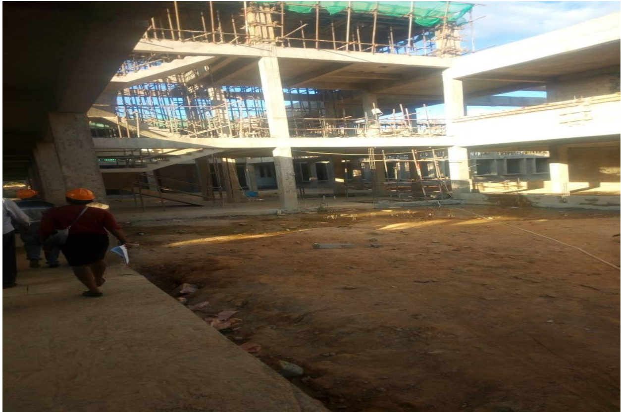
Part of the Chinsali General Hospital toured by your Committee
