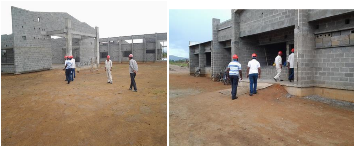
Construction of the administration block and outpatient department at Muyombe
